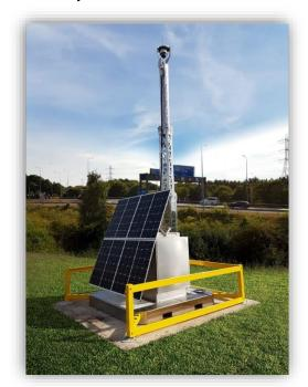
To overcome these challenges, Kier Highways proposed to design and build a Solar IP CCTV System (SICS) which could be quickly and easily deployed to locations without power or communication infrastructure.
